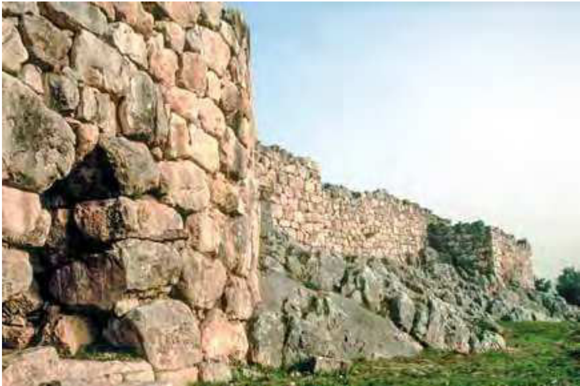
Photo of the west side of the citadel of Tiryns. The right angles and clean break lines in the bedrock show that the construction site also served as a quarry.
